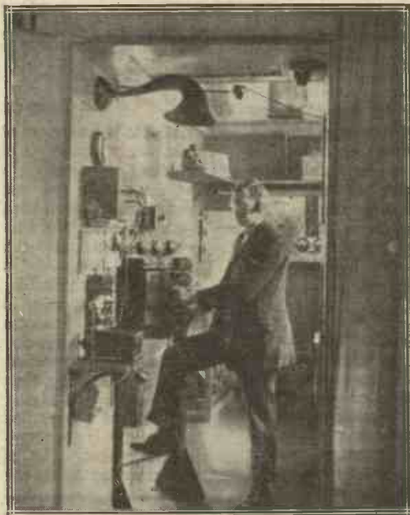
The controls being carefully adjusted at the Zurich Station.
